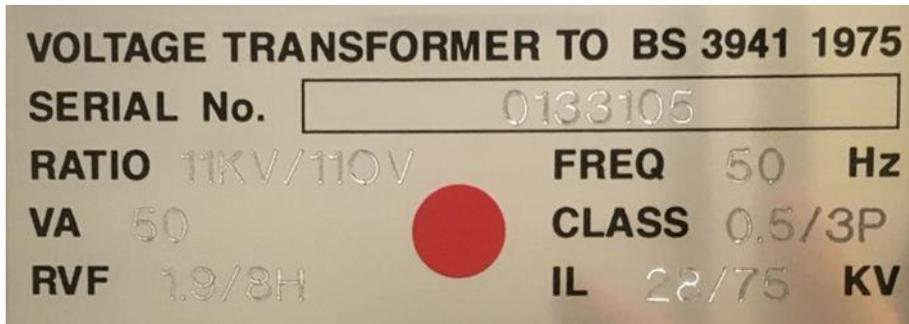
Where in the example the ratio is 11kV/110V; the rated burden is 50VA; the accuracy class is 0.5/3P<sup>7</sup>; and the serial number is 0133105.
